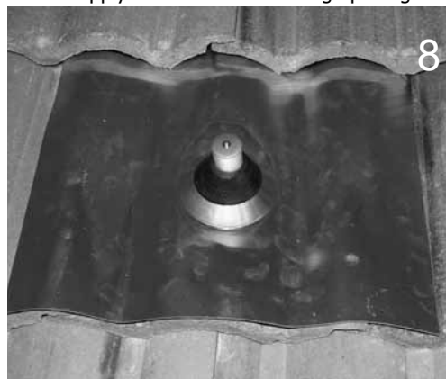
8 Pre bend the flashing to follow the contour of the tile if curved. Install counter flashing collar.
