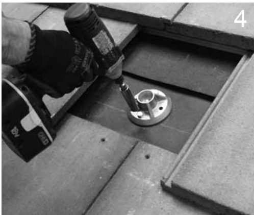
4 Align Q Base over rafter center and drill 2 each 7/32" pilot holes. Place grade 8 Machine Bolt under Q Base in hex slot, threads pointing up. Lag Q Base into Rafter on Marks.
