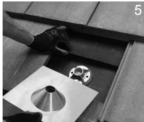
5 Carefully clean the building paper then install Primary Flashing in either a three course method, or properly lapped paper method. Now is a good time to apply sealant to the flashing opening.
