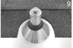
Allow roofing to proceed to the next mount Install counter flashing ring, and rail hardware. Top of Post must be sealed if not installing roof right away.
