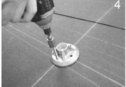
Fill pilot holes with appropriate sealant. Seat Secure post to base plate turning post onto Allow roofing to proceed to the point that the grade 8 bolt through bottom of Q base. Place captive base plate bolt. base plate over drilled holes and secure lags in place, with 15 ft/lbs torque.
